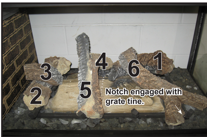
Log Assembly Installed.
