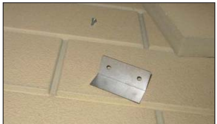
Figure 2 Stone Retainer and Screw
