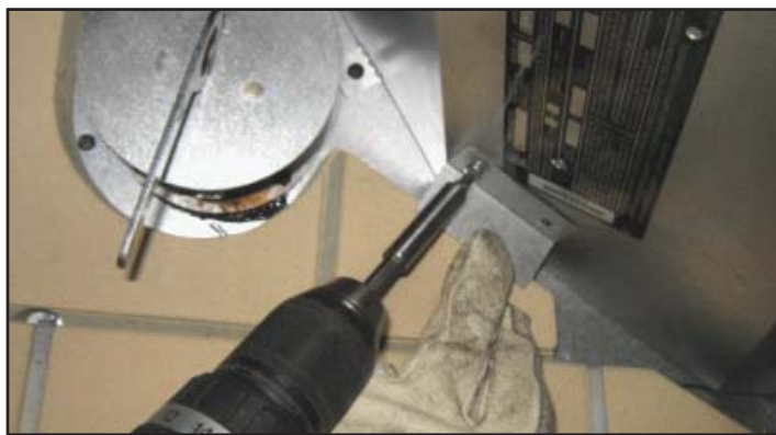
Figure 8 Attach Retainer
