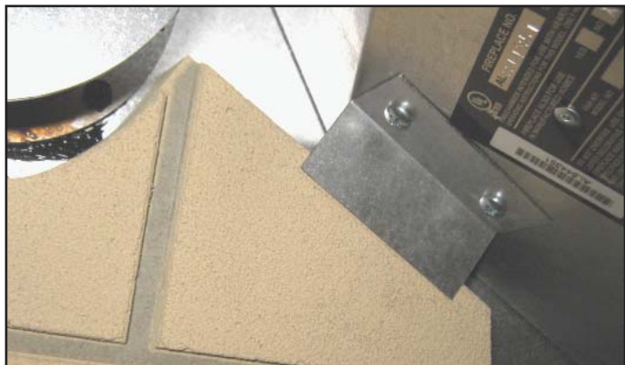
Figure 9 Retainer Installed
