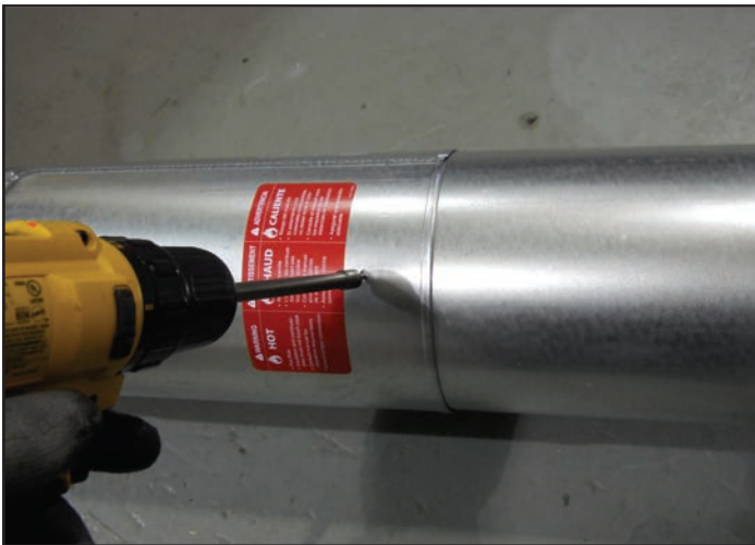
Figure 7.4 - Screws into Slip Section
