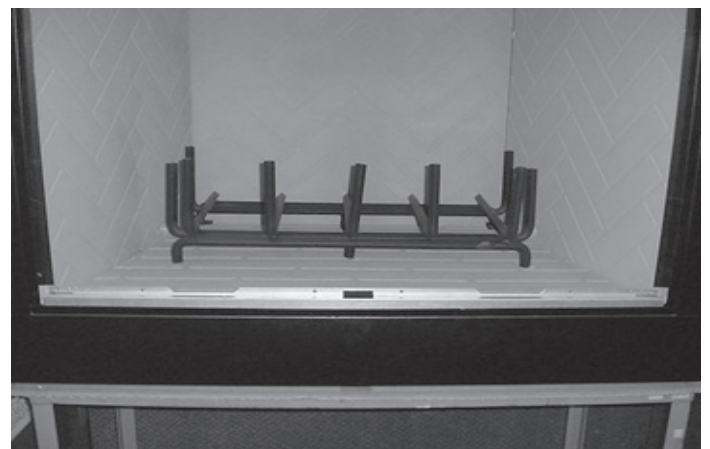
Figure 2 - Installed Door Track
