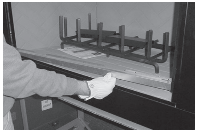
Figure 1 - Install the Door Track
