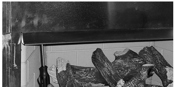
Figure 3 Remove 3 Screws
