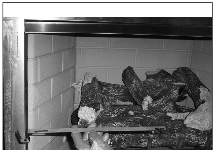
Figure 4 Install Upper Left Bracket
