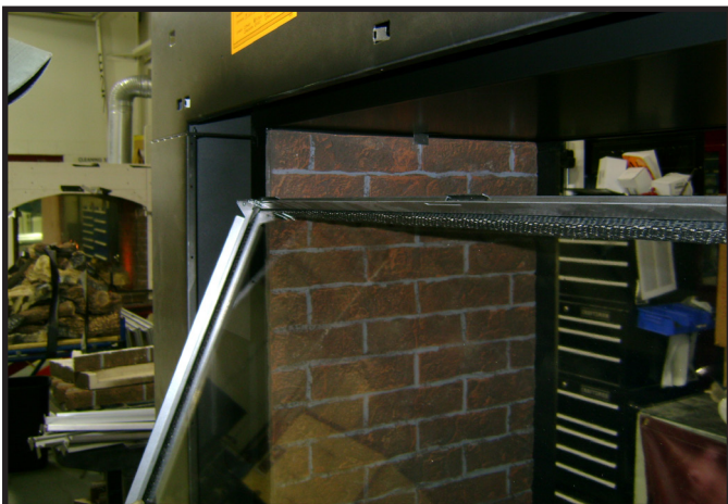
Figure 11.2 Initial Positioning of Frame into Opening.
