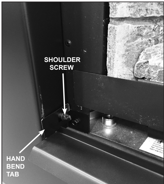
Figure 7 Hand Bend Tab & Shoulder Screw
