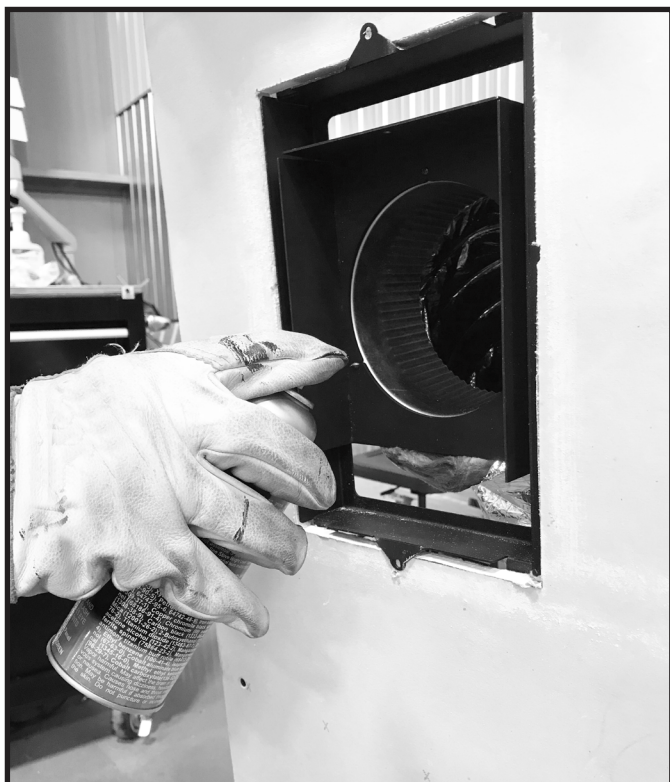
Figure 6.4 Paint Outer Wrapping of Flex Vent (Optional)
