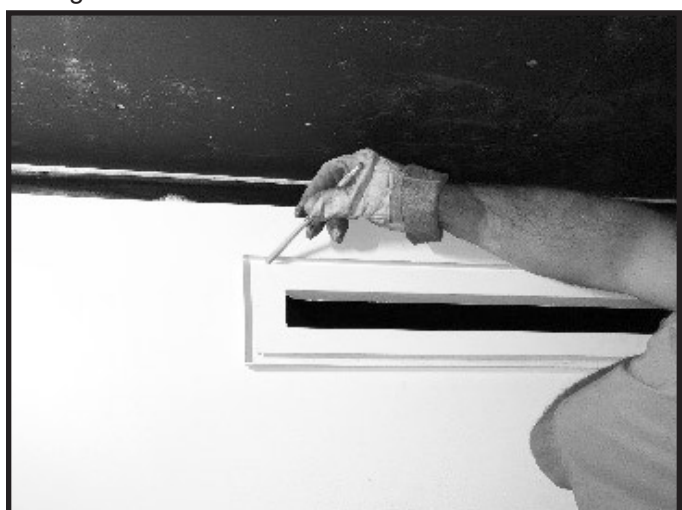
Figure 3 Mark Holes for Register Backer
