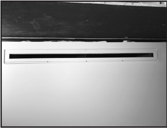
Figure 6 Register Cover Installed
