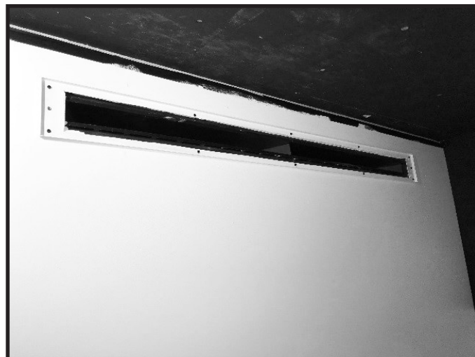
Figure 4 Register Backer Installed
