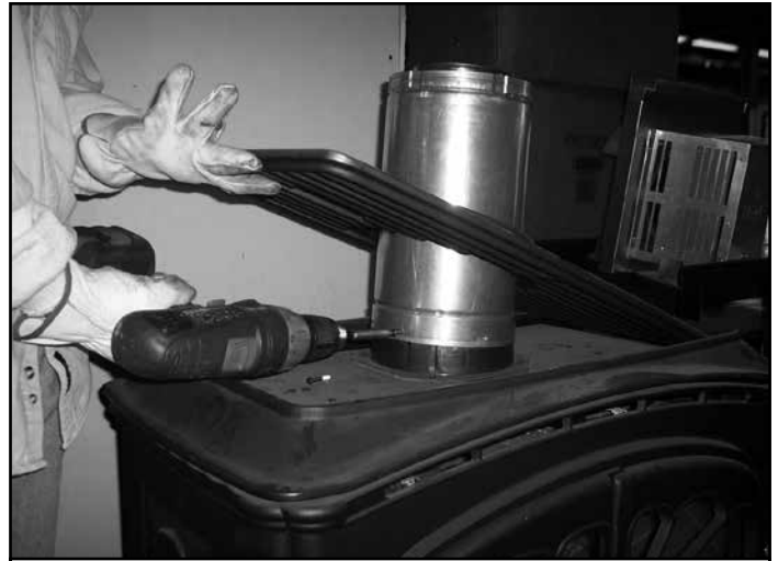
Figure 7 Fasten SLP Vent to Stove
