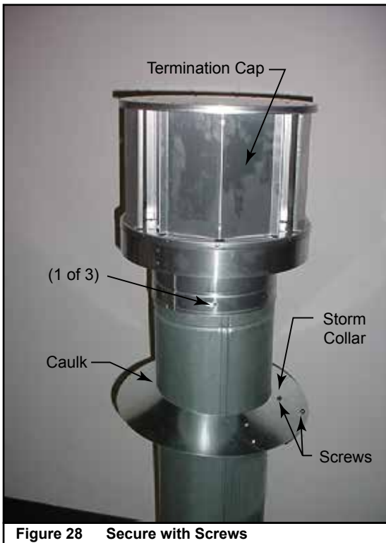
Figure 28 Secure with Screws
