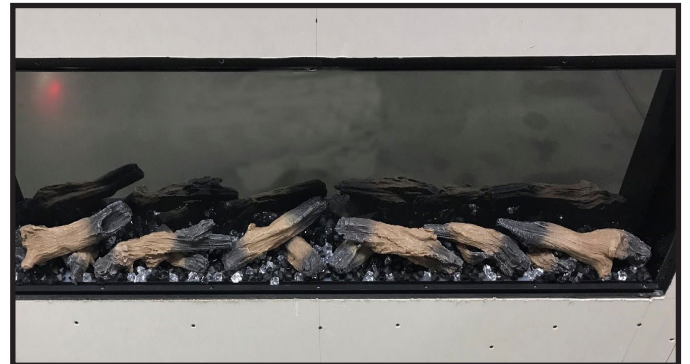
Figure 4.11 Larger Log Installation
