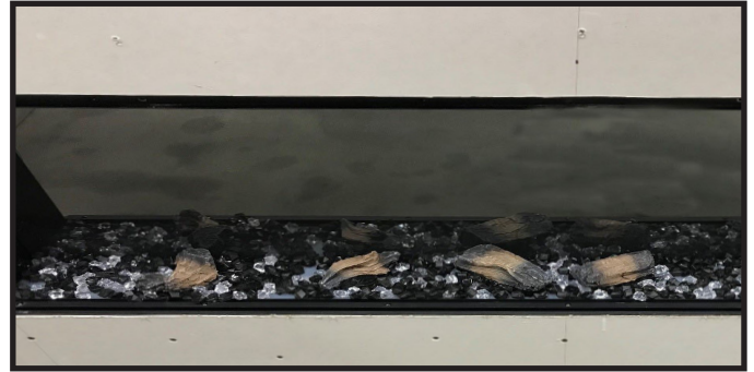
Figure 4.10 Media and Small Logs Installation
