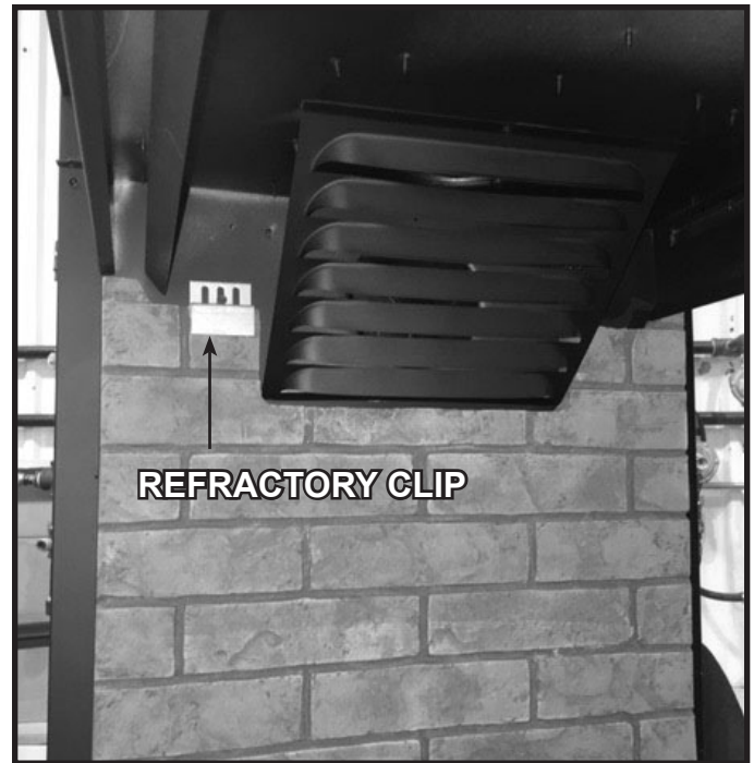
Figure 5. Refractory Installed (Exhaust Side)
